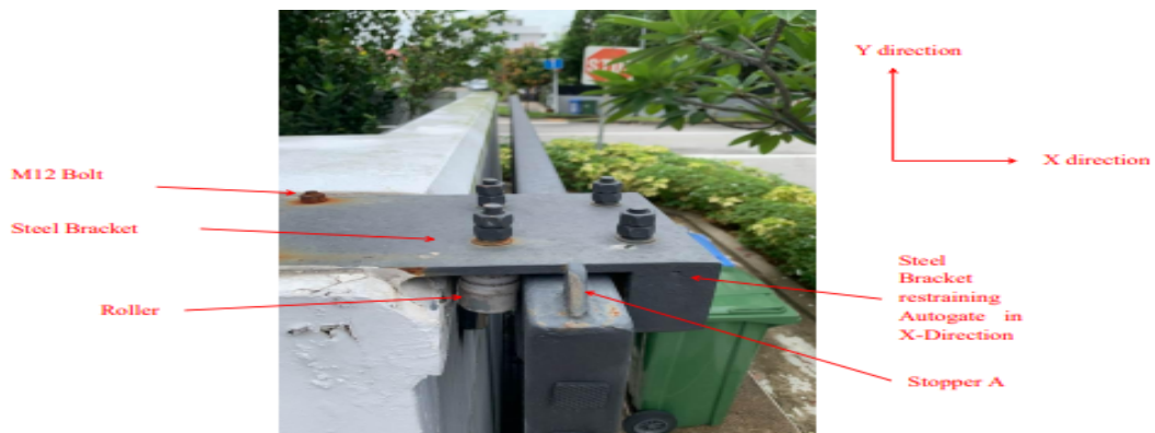
Photo 29. Plan view of Steel Bracket and top frame of Autogate. Steel Bracket is to restraint the Autogate in the X-direction, Stopper A & B are to restraint the Autogate in the Y-direction
